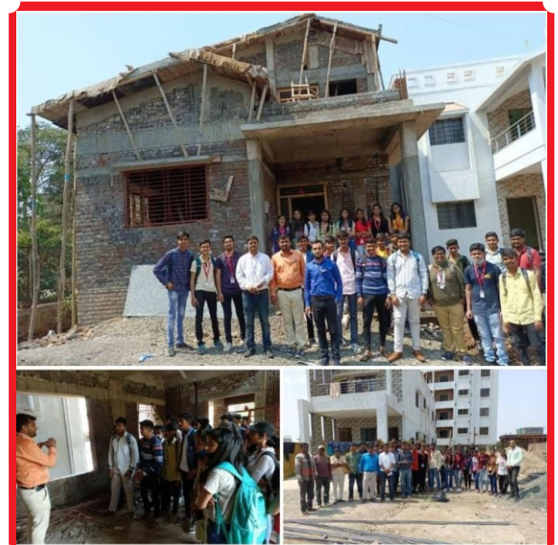
Students of Civil Engineering at Construction site
