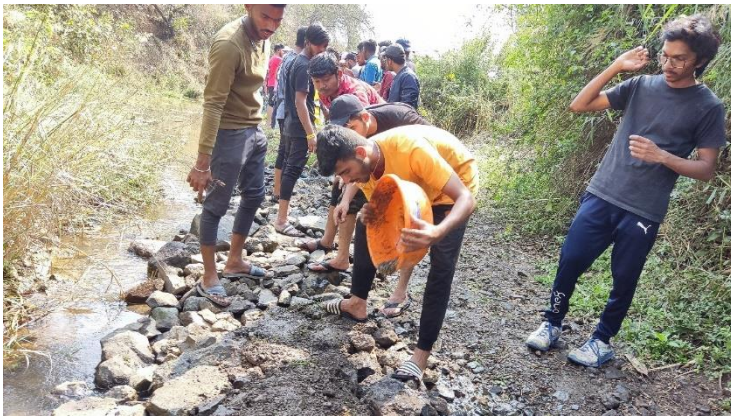
Construction of "Pai Vat"
